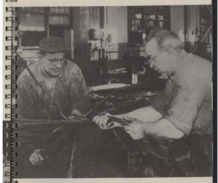
Above: Highly skilled splicers fashion fatigue resisting splice. Here they are splicing a boom support to be used on one of the gigantic shovels which will dig high-grade iron ore from one of the United States Steel Corp. mining operations.
