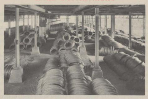
High carbon rods received in open gondola railroad cars from American Steel & Wire South Works, Worcester, Massachusetts, picked up by overhead monorail crane, using hair-pin hook, and placed in storage according to type stock and heat number.
