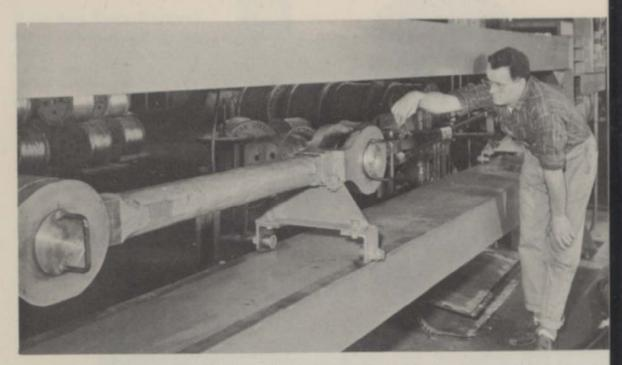
The lives of pilots are at stake when these slings are used in launching planes from the decks of carriers. Here is shown the rigid test by skilled men and special equipment and the certified sling being packed for shipment.
