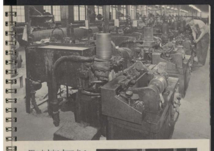
Wire is being drawn in a liquid solution which acts both as a lubricant and as a means of dissipating heat. Both tungsten carbide and diamond dies are used in this operation. Wire in photograph is being drawn directly onto 25 pound spools for stranding in the rope mill.
