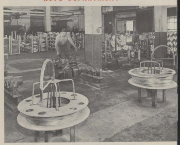
Wire placed on various size spools depending on the size of wire and spool capacity of the machine which will strand it. Mechanism in foreground is "dead pay-off" (designed at New Haven Works), so named because the coil remains motionless and wire is uncoiled by gooseneck in center. Here, constant vigilance is required to assure wire goes on spools in uniform layers under proper tension.
