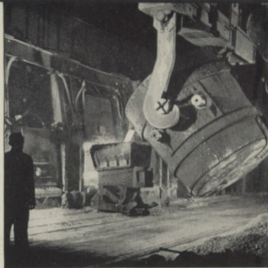
POURING MOLTEN IRON INTO OPEN HEARTH
