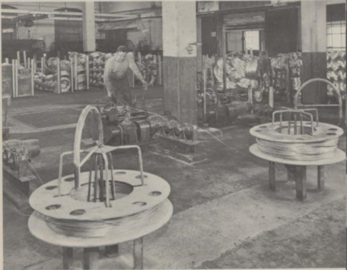
Wire placed on various size spools depending on the size of wire and spool capacity of the machine which will strand it. Mechanism in foreground is "dead pay-off" (designed at New Haven Works), so named because the coil remains motionless and wire is uncoiled by gooseneck in center. Here, constant vigilance is required to assure wire goes on spools in uniform layers under proper tension.
