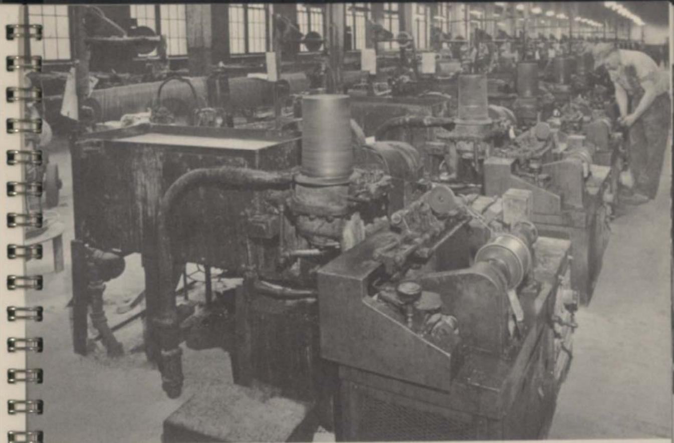
Wire is being drawn in a liquid solution which acts both as a lubricant and as a means of dissipating heat. Both tungsten carbide and diamond dies are used in this operation. Wire in photograph is being drawn directly onto 25 pound spools for stranding in the rope mill.
