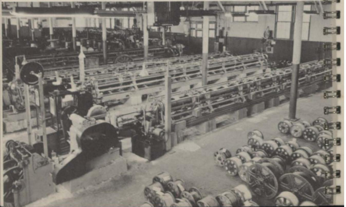
Here operator is about to load a 500 pound spool of wire into a strander. Spools are suspended in cradles, one behind the other. Wires are strung through a long tube. Strand is then formed by twisting these wires. The major portion of strand produced, as shown below, is further processed into wire rope. Some machines run in tandem are capable of twisting 48 wires around a center wire to form a 49-wire strand.
