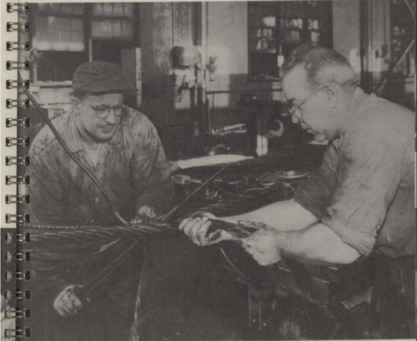
*Above:* Highly skilled splicers fashion fatigue resisting splice. Here they are splicing a boom support to be used on one of the gigantic shovels which will dig high-grade iron ore from one of the United States Steel Corp. mining operations.
